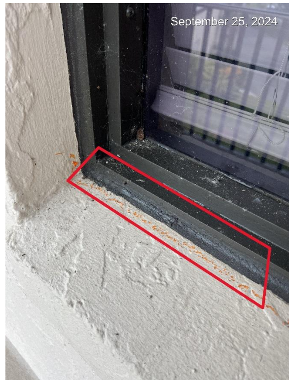
Figure 7. Example of Failed Sealant.
