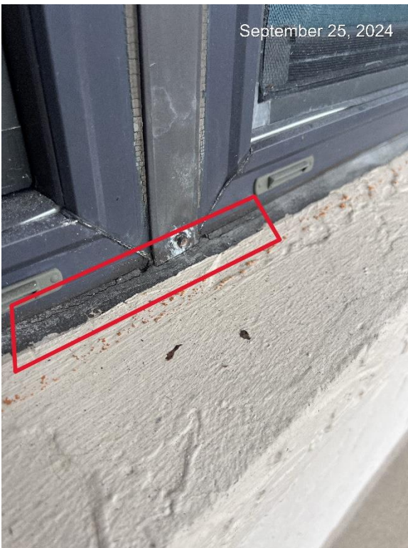
Figure 6. Example of Failed Sealant.
