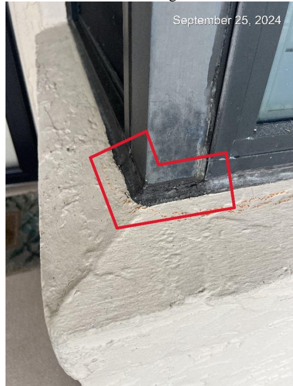
Figure 5. Example of Failed Sealant.
