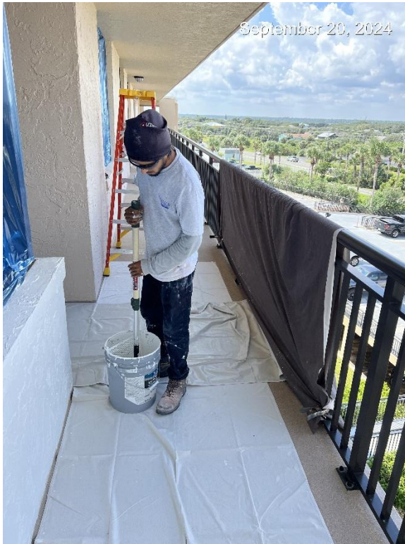
Figure 1. Primer application on the 4 th Floor Walkway.
