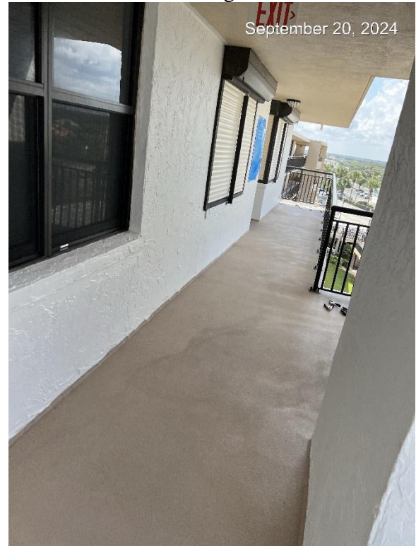
Figure 2. North Side of 4 th Floor Walkway Primed.
