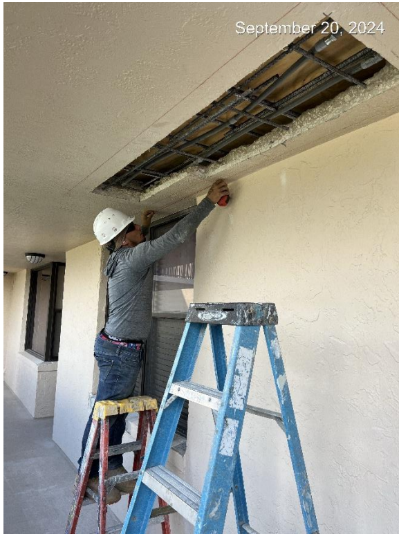
Figure 4. Employee Preparing to Form a Full Depth Repair.
